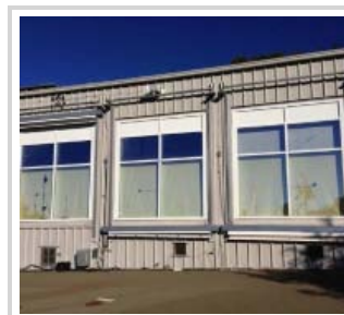
Outdoor view of the windows tested facility. Click to enlarge.
