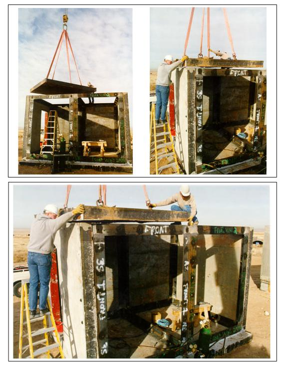
Figure A.3. Placement of the South Bay Structure roof panel (3M PREP 20.tif, 3M PREP 19.tif, 3M PREP 17.tif).
