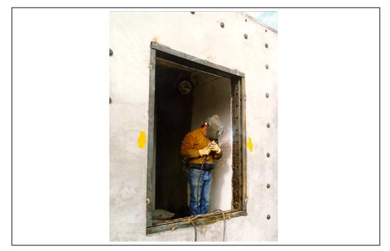
Figure A.6. View of a technician welding the window frame to the embed (3M PREP 12.tif).
