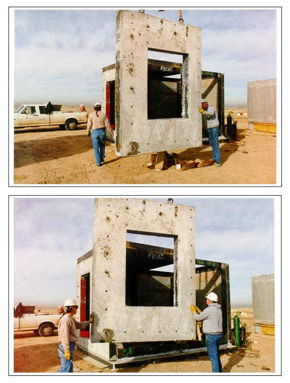
Figure A.5. Placement of the South Bay Structure front panel into the modular structure steel frame (3M PREP 03.tif, 3M PREP 04.tif).
