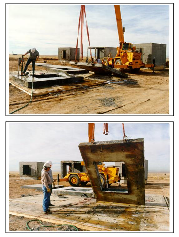
Figure A.4. Views of a crane lifting the South Bay Structure front panel (3M PREP 16.tif, 3M PREP 01.tif).
